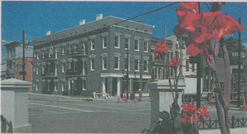
The Hummel Building at 1401 Elm St. was built in 1878 as a mixed-use development, with multifamily housing, a market and saloon.
